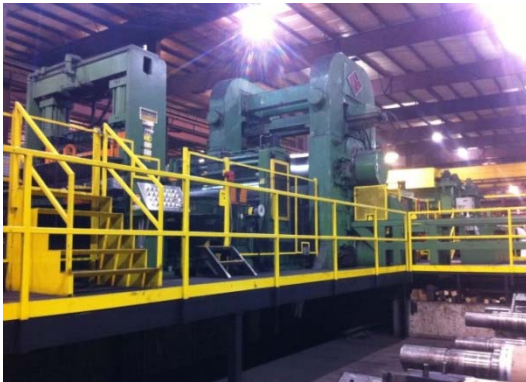
Side View of Cold Rolling Mill
